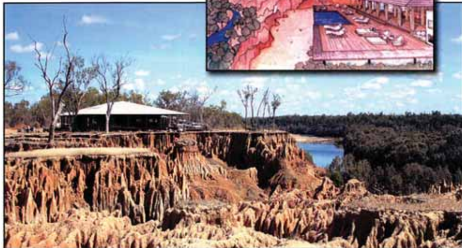
Resort under construction overlooking the Mitchell River. INSET: Artist's impression of Wrotham Park Station.
