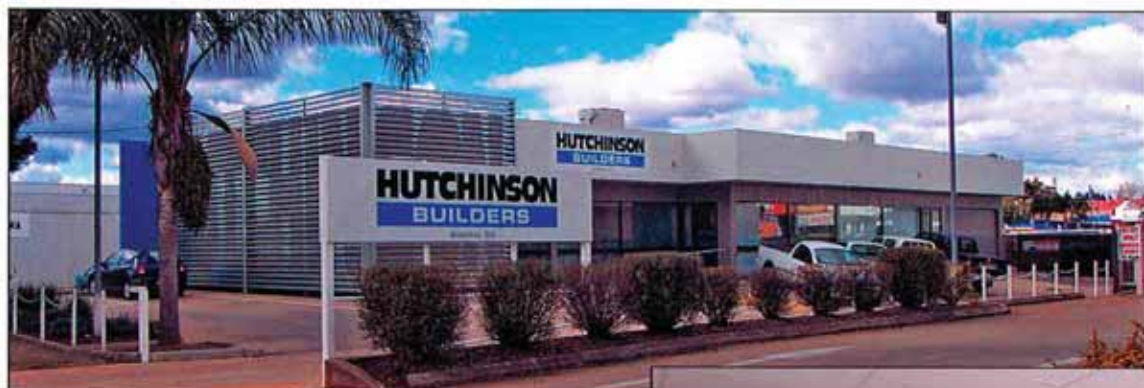
LEFT: Hutchies' new office in Toowoomba with its eye-catching Hutchinson sign.
